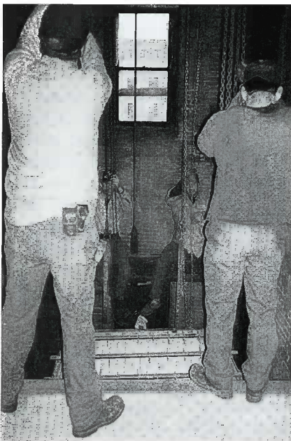
Hoisting the kiln—1 centimeter per pull.
